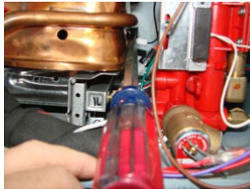
Sometimes the electrode may be arcing to the manifold preventing ignition. If this appears to be the case a screwdriver can be used to gently reposition the electrode away from the manifold.
