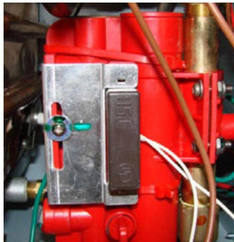
Proper setting for operation. Notice the screw is approximately 2/3 of the way up the slot.
