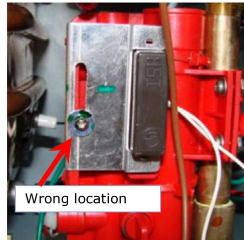
This example is too high notice the screw is located at the bottom of the slot. This location could cause the unit problems with operation.
