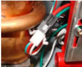
Find the wire harness connection for the blower and verify it is plugged in properly.
