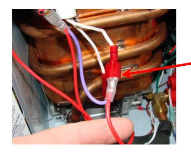
Terminal for the cold weather t-stat circuit.
