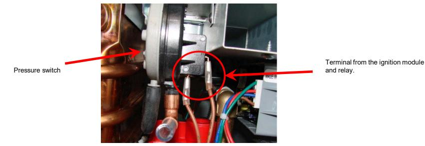
This switch is a normally open contact that closes when a vacuum is created by the operation of the blower motor. This causes the switch to close allowing power to pass to the ignition module and operate the gas valve. If these terminals are not installed attached to the switch the motor would still operate, but the gas valve would not.
