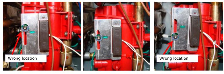
This example is too low notice the screw is located at the top of the slot. This location could cause problems with operation.
