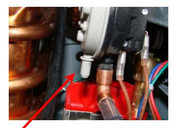
If the hose is not connected here or at the blower housing then the heater cannot close the switch and will not ignite.
