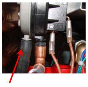
This is the tube that connects the pressure switch to the blower housing. Even if this hose is securely in place still take time to look for wear or possible leaks.
