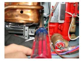
Sometimes the electrode may be arcing to the manifold preventing ignition. If this appears to be the case a screwdriver can be used to gentle reposition the electrode away from the manifold.
