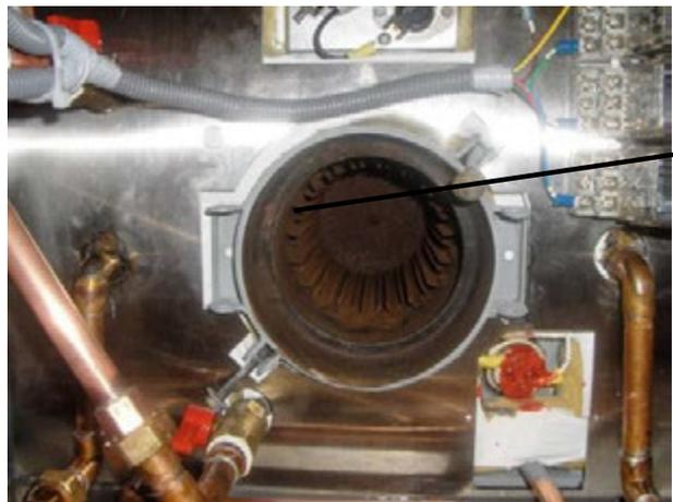
2. Once the combustion chamber has been removed. Use a long handled wire brush, and brush the heat transfer tabs, to loosen soot deposits. Failure to do so will reduce the Aqua-Hot's heat transfer capabilities.
