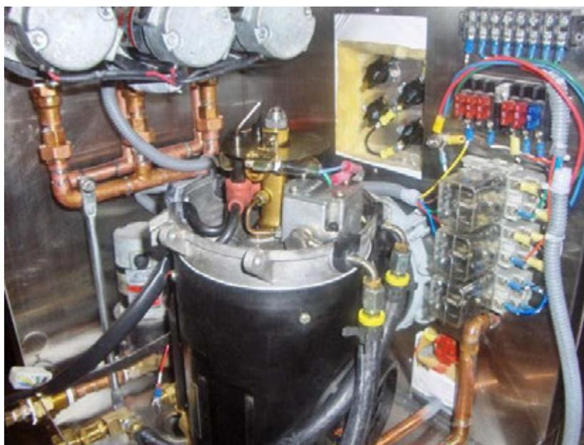
2. Carefully pull the Diesel-Burner away from the Aqua-Hot 4 to 5 inches before rotating the burner, and then remove.
