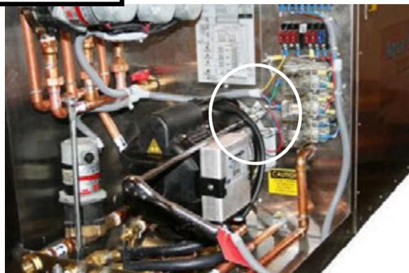
**NOTE: When reinstalling the diesel burner be careful not to damage the photo disc or bend the electrodes. Also, be careful to not pinch any wires between the burner and the Aqua-Hot Tank.**
