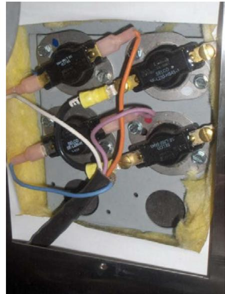
1. Disconnect the thermostat wires by firmly pulling on the pink connectors. Remove the wires from the wire access slot.
