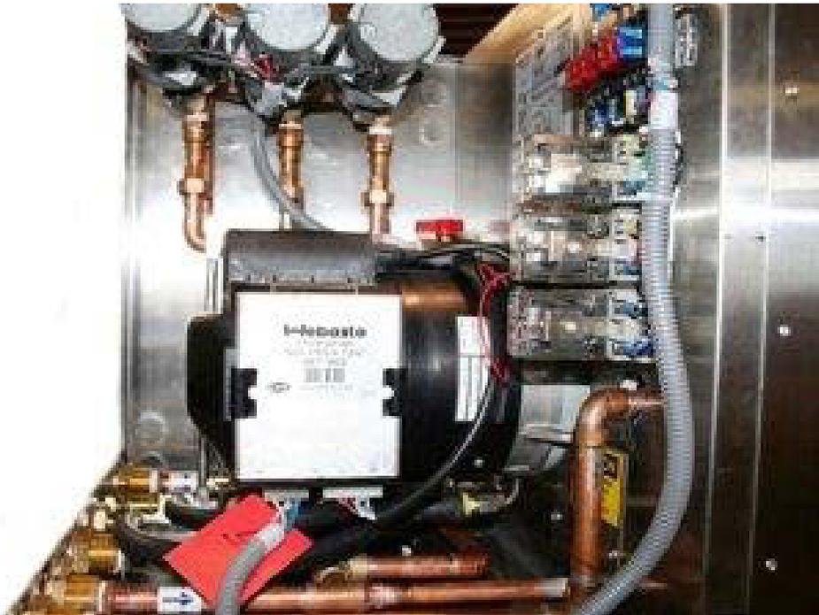
1. Locate the Diesel-Burner's Controller and connect both plugs.
