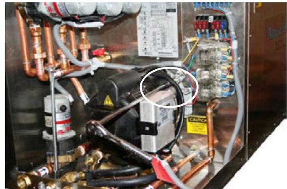
3. The Diesel-Burner is secured to the Aqua-Hot with two nuts that can be loosened, and swung out of the way by using a 10mm socket wrench with a 10 inch long extension.
