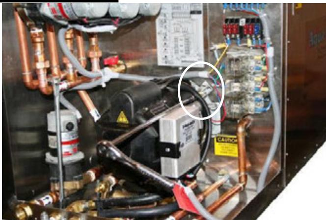
1. The Diesel-Burner is secured to the Aqua-Hot with two nuts that can be loosened, and swung out of the way by using a 10mm socket wrench with a 10 inch long extension.
