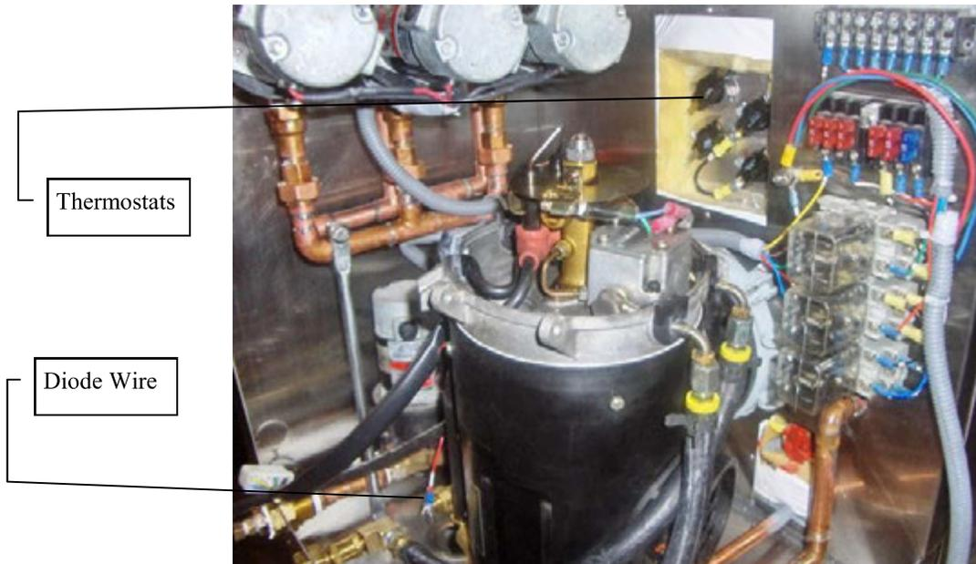
4. Carefully pull the Diesel-Burner away from the Aqua-Hot 4 to 5 inches before rotating the burner, and then remove.
