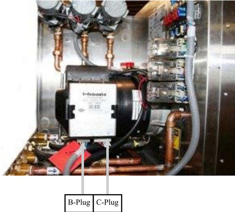
1. Locate the Diesel-Burner's Controller and disconnect both plugs.
